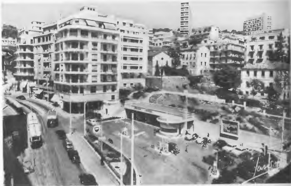
Algier - Rue Michelet. Station service BP
